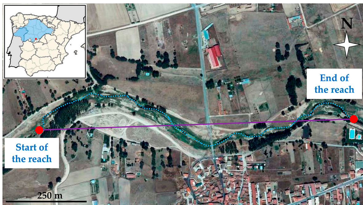
Figure 1. Top left view: Duero River basin and case study situation (source Duero River Basin Authority). Detailed view: Analyzed reach (Digital orthoimage from National Plan for Territory Observation [61]). Coordinate Reference System: EPSG: 25830.
