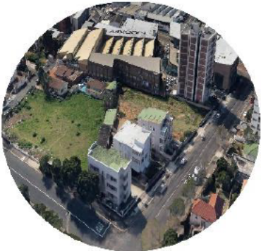
Figure 8.13. image showing aerial view of site. (source: Google earth)
