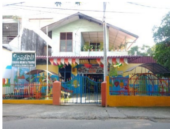
Figure 1: RA Al Ittihadiyah Building
