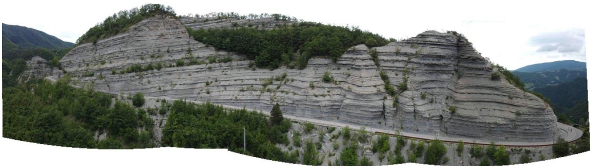
Figure 82. Panorama built with Photoshop using the aerial pictures taken during the inspection of May 2020
