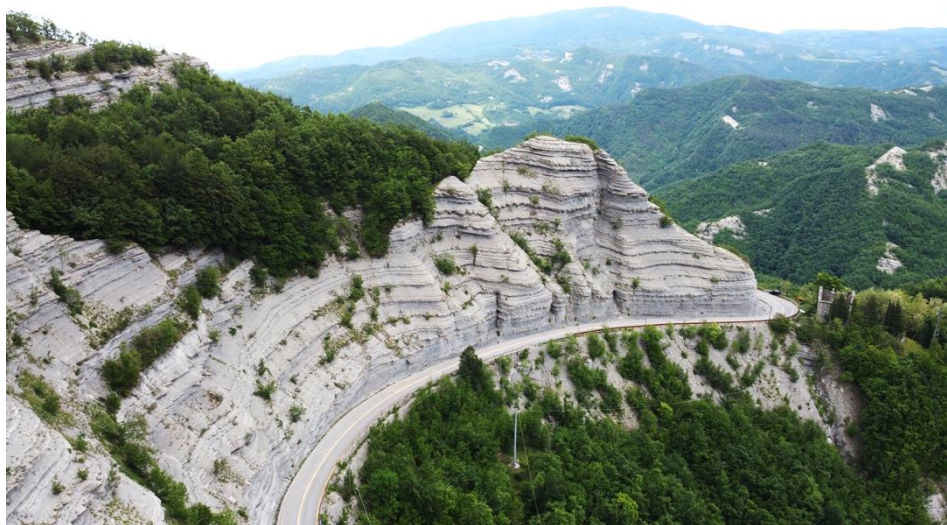
Figure 80. Aerial view of Le Scalacce during the inspection in May 2020
