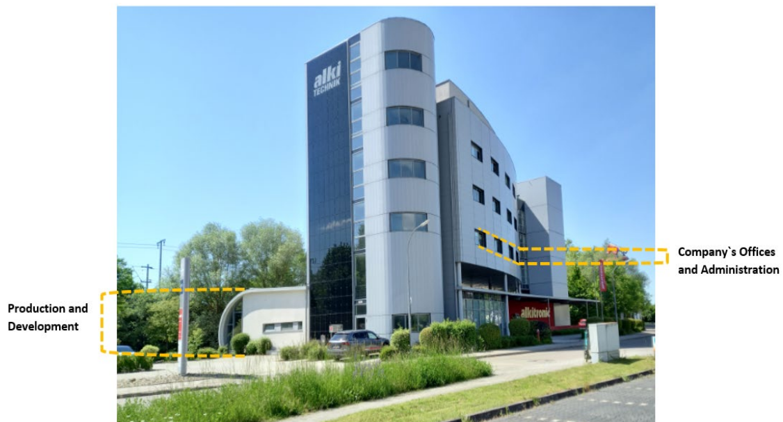
Figure 5 - View of the company facilities.
