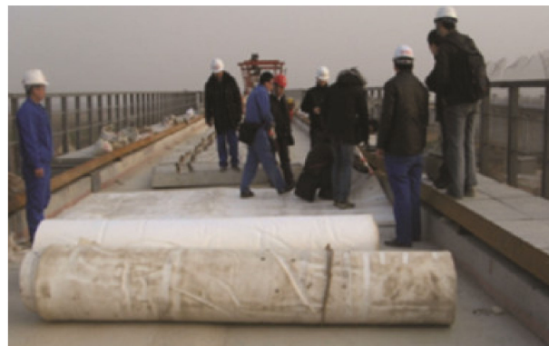
Figure 2. Installation of ballast mat.
