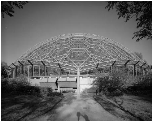
Imagem 24 - Climatoffice, Dome Geodésico, no Jardim Botânico de Missouri, St. Louis Climatron, Buckminster Fuller e Norman Foster, 1971. Imagem retirada no dia 11.07.2021 do site: https://upload.wikimedia.org/wikipedia/commons/1/11/Climatron%2C_WEST_SEGMENT_HABS_MO%2C96-SALU%2C105L-3.jpg ou https://www.britannica.com/biography/R-Buckminster-Fuller
