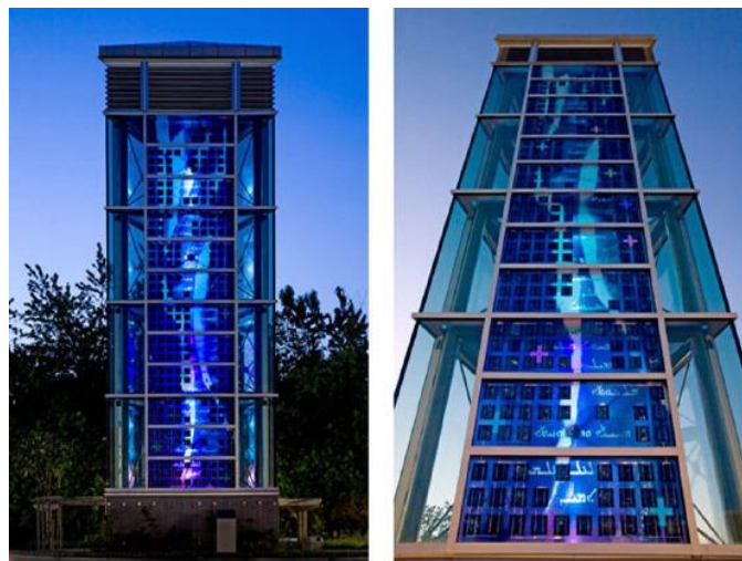
Figure 2-87. Lux Nova . Sarah Hall. 2007. Wind tower Regent College, Vancouver, Canada. ©Stained Glass Peters GmbH.
