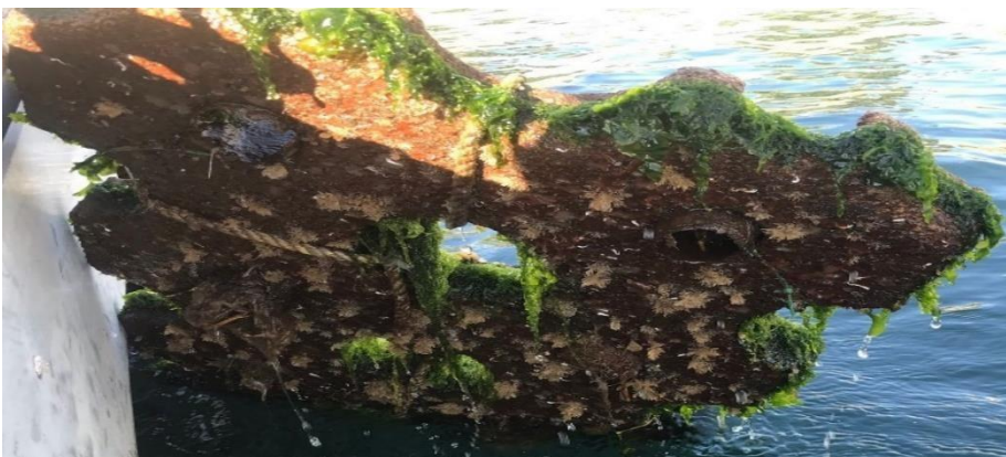
Figure 29: Mussels and algae attached to the Floating Wetland Island platform.
