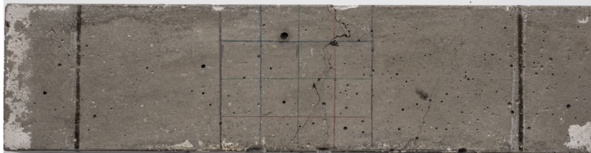
FIGURE 5.6: Localised macro-crack observed in specimen 3.0%-400-2.
