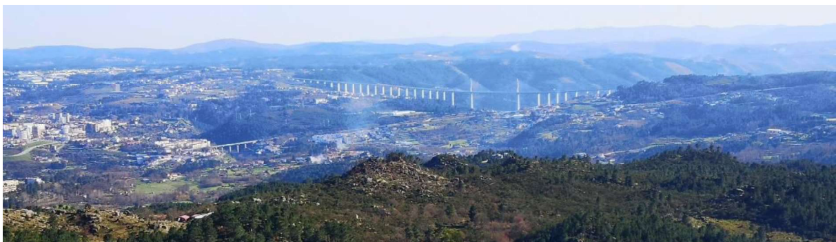
Fig. 2 – Panoramic view of sector III from the Occidental Mountain Range (Alvão Mountain). High Plateau (MPNP) well preserved contrasting with the entrenched valley of Corgo River, a tributary of Douro of the right margin. Upstream of the minor bridge at left, there is the migration of the erosion wave and the transient knickpoint locate at the city of Vila Real.
