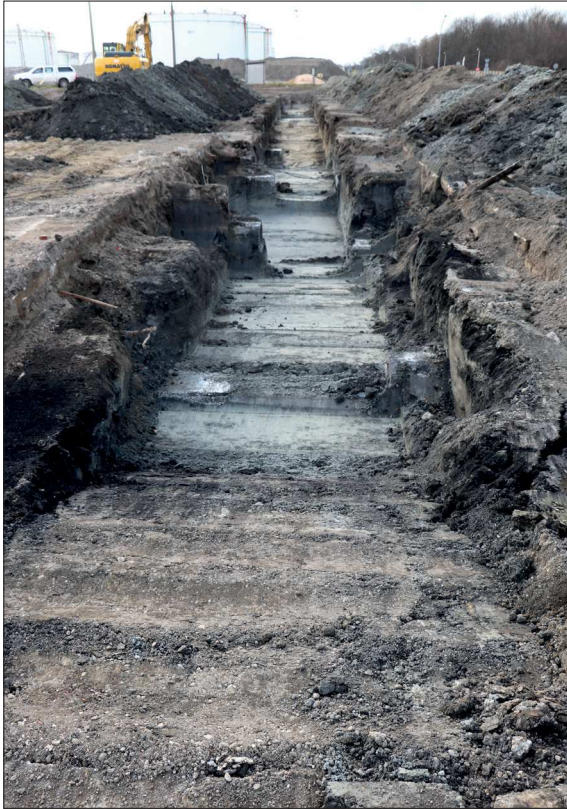
Fig. 2. Excavation circumstances at the RepCat area (Photo: Bence Simon).
