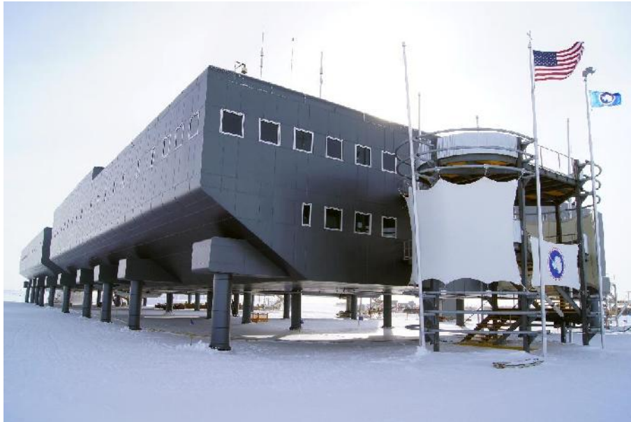
Figure 3-12 Amundsen-Scott South Pole - Entrance 157 (courtesy National Science Foundation)
