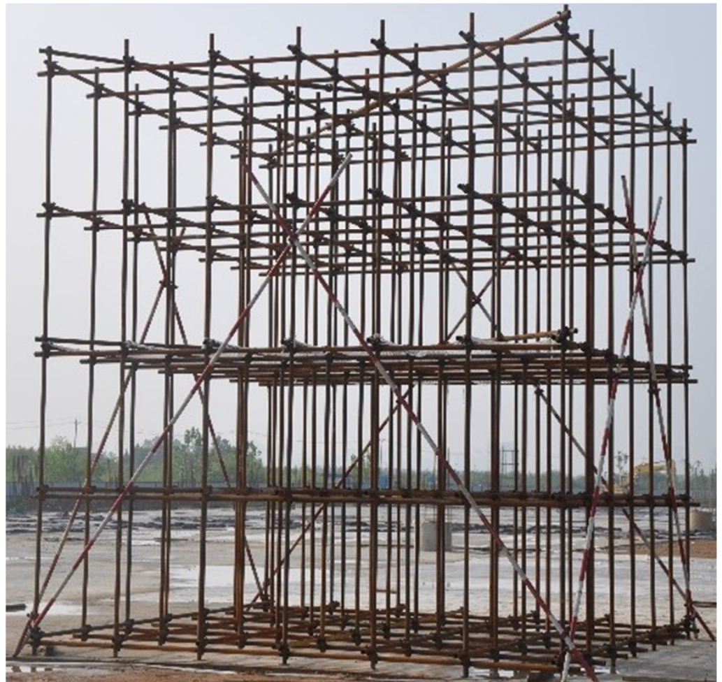
Figure 20. The photography of the high formwork.
