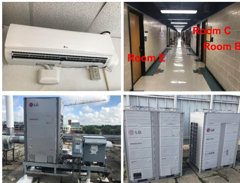
Figure 2-3 Pictures of Indoor and Outdoor Units
