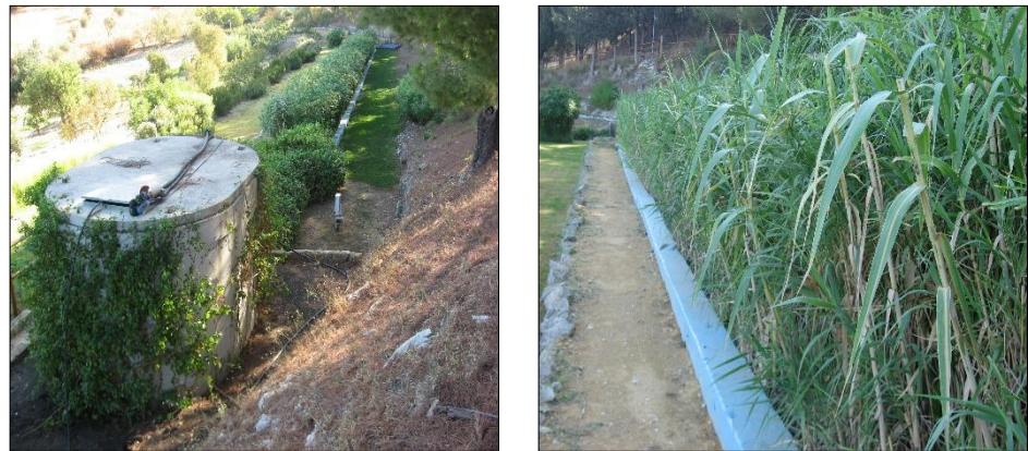
Figure 2. A view of the pilot-scale horizontal sub-surface flow systems (HSSFs) constructed wetland CW.
