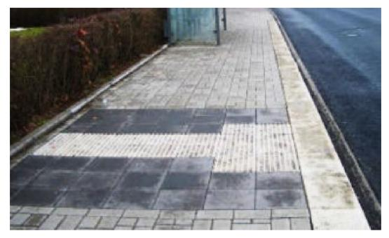
Figure 6. The layout of tactile surfaces on a bus stop platform in Germany. Source: Own elaboration
