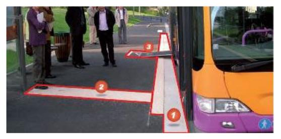
At a bus stop, the blind or visually impaired traveller should be able to identify the position of the vehicle's front door to be close enough to hear the announcement of the line and destination indication (which the fleet of vehicles provides) and be in verbal contact with the driver (CERTU, 2010).
