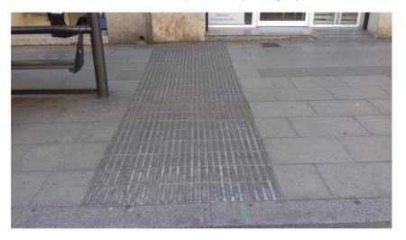
Figure 8. The layout of tactile surfaces on a bus stop platform in Spain. Source: Own elaboration
