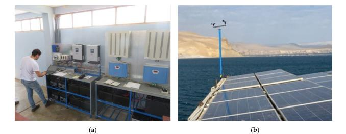
**Figure 5.** (a): Overview of the inverters, controls, and battery consoles of the Laguna Grande microgrid, (b): view of the rooftop-mounted PV array with the anemometer and wind vane in the background.
