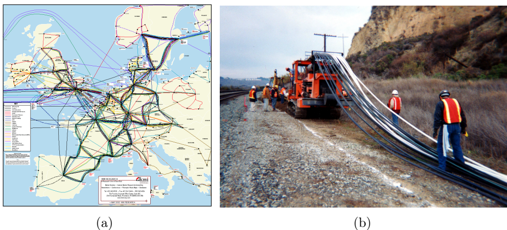
Figure 7.1: Terrestrial Fiber-optic network (a) and examples of infrastructure installation (b). Source: [68] [69]
