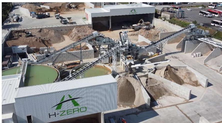
Figure 1. CDW recovery plant to water-washed recycled aggregate [35].
