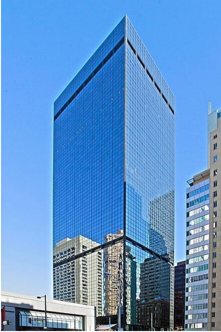
e) 555 Office Building Building Reference: Pre-1980 Construction Year Built: 1978 Building Height: 40 Stories Façade Materials: Glass
