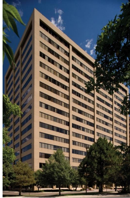
j) Stanford Place III Office Building Building Reference: Post-1980 Construction Year Built: 1986 – Renovated in 2017 Building Height: 17 Stories Façade Materials: Brick, Glass
