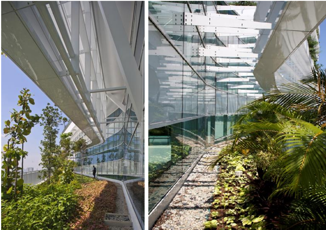
Figure 3.12: Psychological benefits of increased plant visibility as visual comfort, as well as shading advantages from using vertical greenery systems on the Solaris office buildings façades.
