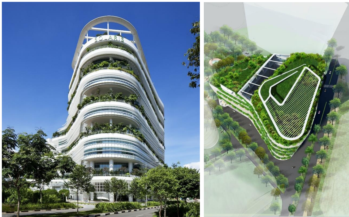
Figure 2.25: Solaris, Singapore, Yeang's own project.
