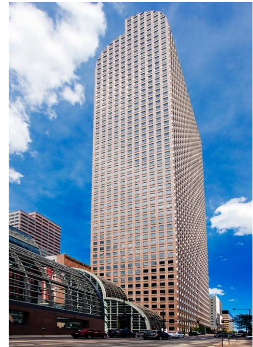
h) Wells Fargo Office Building Building Reference: Post-1980 Construction Year Built: 1983 Building Height: 52 Stories Façade Materials: Red granite, Glass façade
