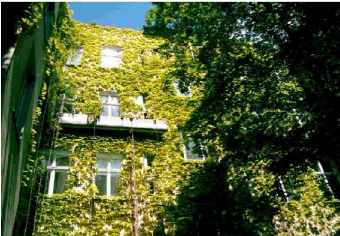
Figure 4.1: In the course of a restructuring of a 100-year-old apartment block, the project "Paul Lincke Ufer" green façade in Berlin, started in 1984. Hanging planting boxes and ivy from Boston were planted in the small inner courtyard to transport much of the vegetation.
