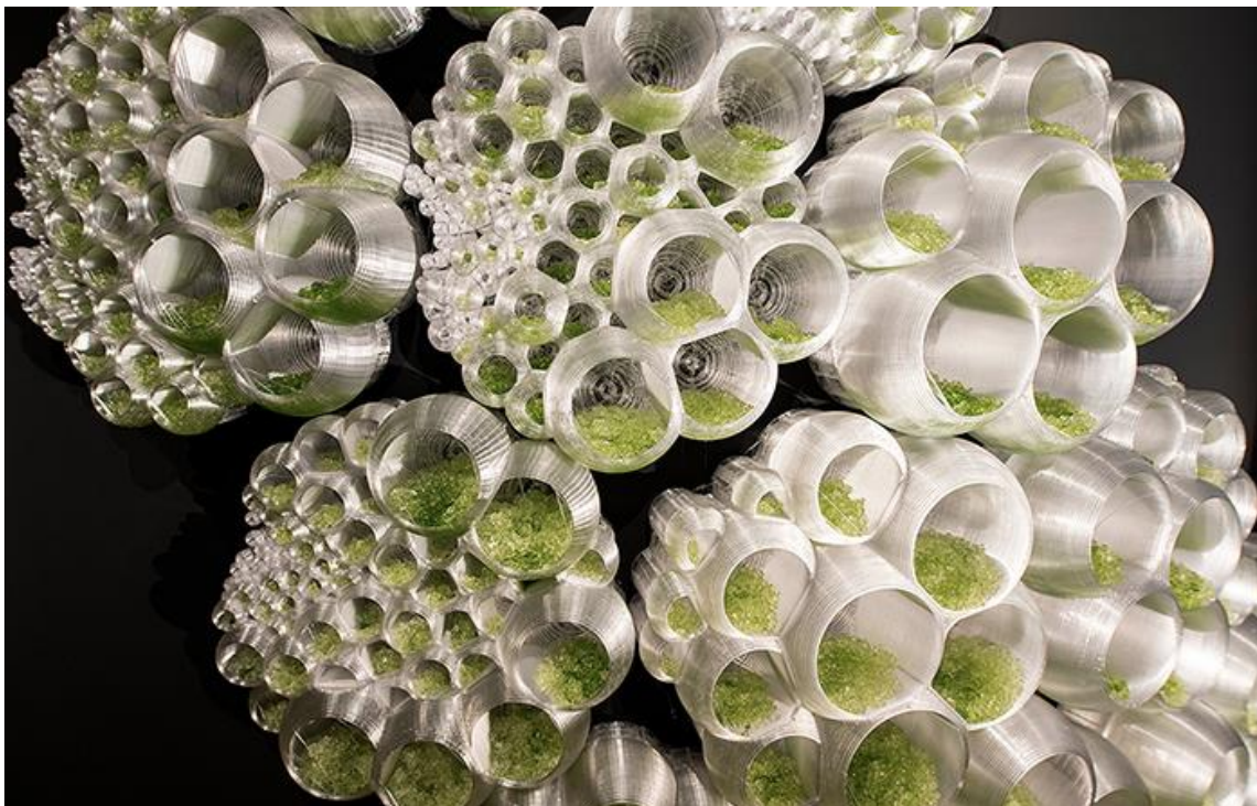
Figure 5.9: Close view of bI.O.serie project which showed details of substrate that consists of porous wall mounted photo-bioreactors.
