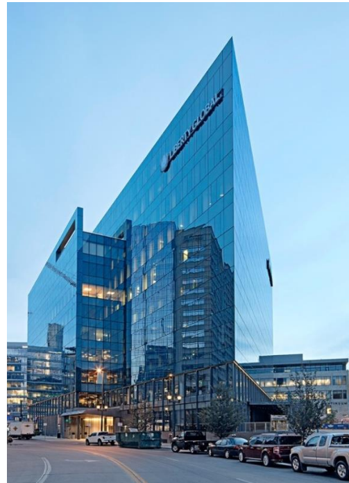
l) The Triangle Office Building Building Reference: New Construction Year Built: 2015 Building Height: 10 Stories Façade Materials: Glass Walls
