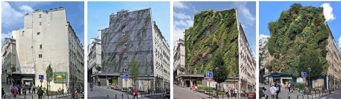
Figure 2.19: Green façade as a vertical greenery system designed by Patrick Blanc in Madrid, Spain.
