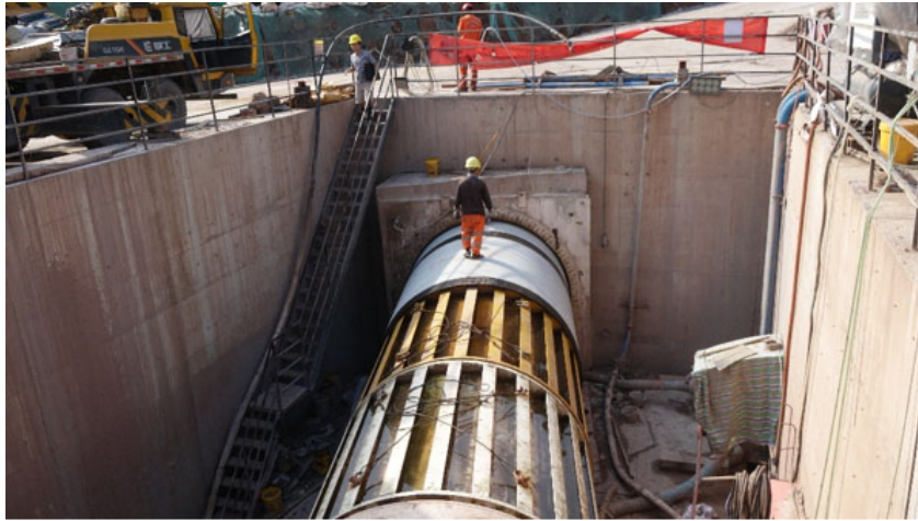
Figure 1 Typical thrust phase of a pipe jacking system
