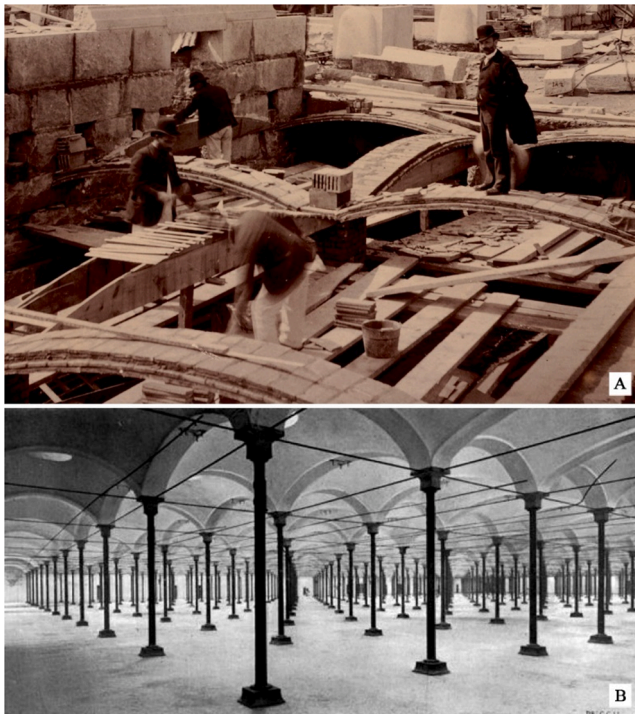
Fig. 1. Example of two buildings with timbrel vaults using thin clay tile. A) R. Guastavino standing on a timbrel arch with the timbrel vaults under construction [Photograph adapted from [31], distributed under a CC BY 2.0 license]. B) Weaving room in Can Batlló industry in Barcelona at the beginning of the 20th century [Photograph by [32], AGDB, Diputació de Barcelona ©].
