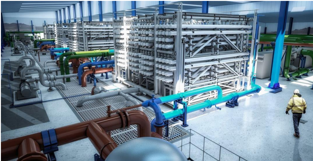
Figure 19: Reverse Osmosis System in Ghana [21]
