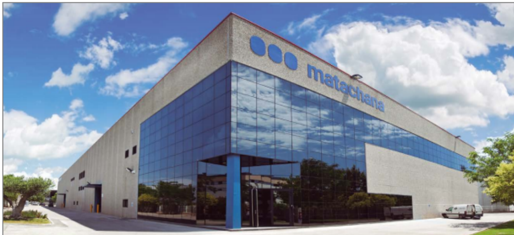
Figure 23. Matachana production center, Castelldefels, Spain.
