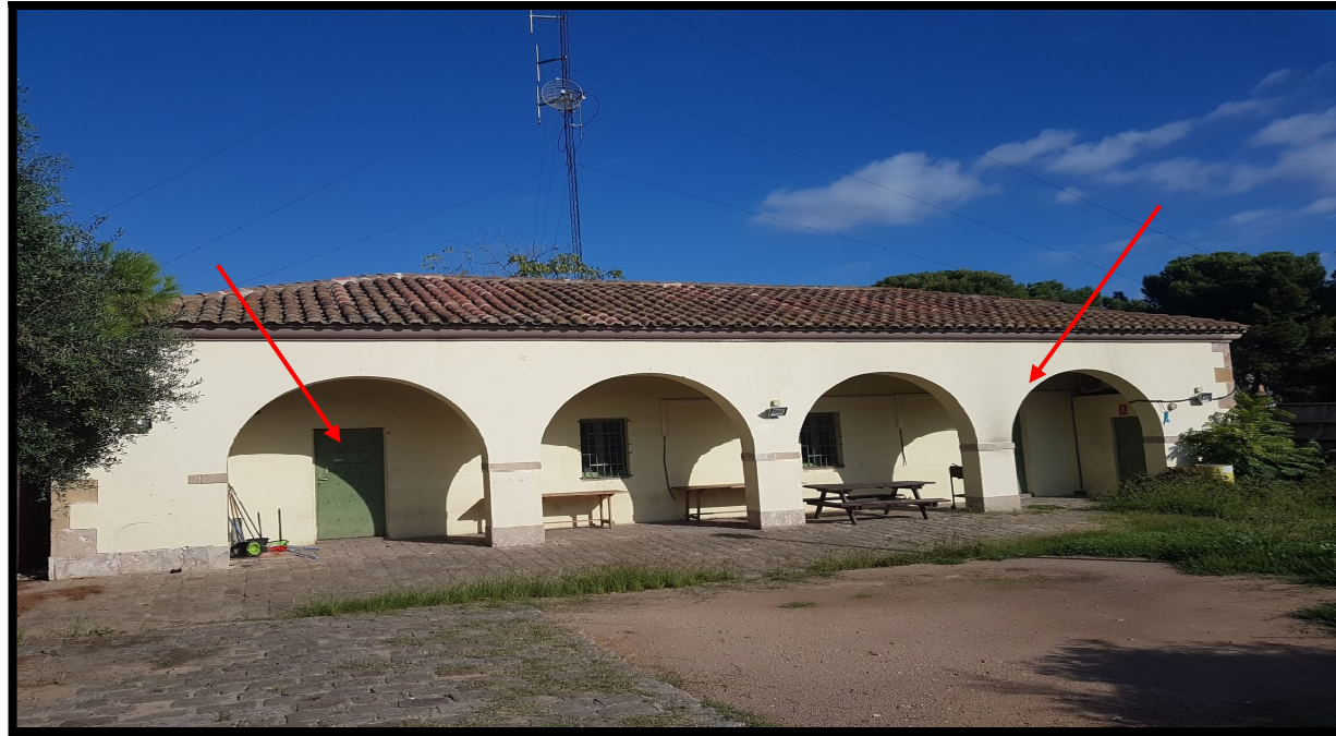
Image: Two accesses to the interior of the building.
