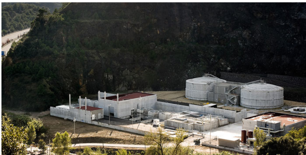
Figure 4.3 Alt Maresme Nord WWTP
