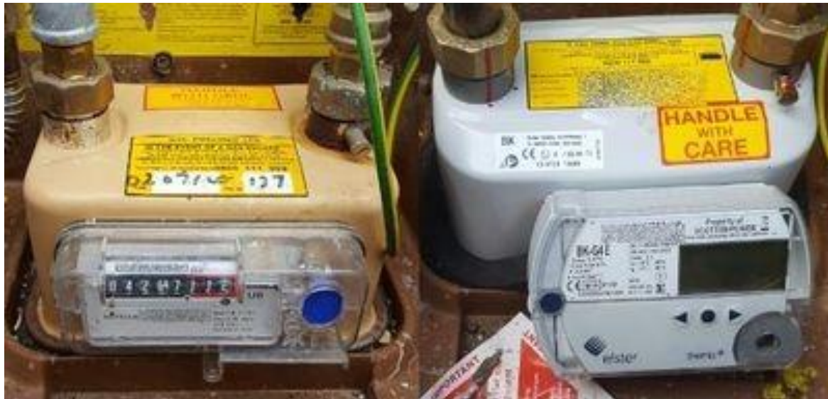
Figure 8. Image showcasing an analogue meter (on the right) a smart meter (on the left) 9
