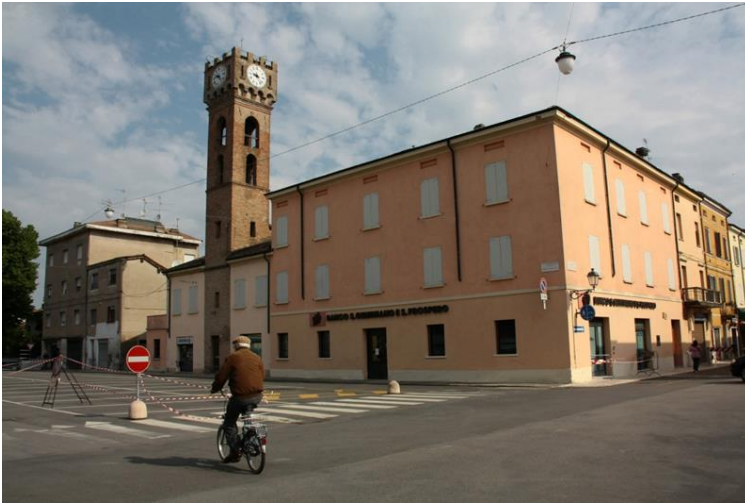
Fig.5. The Clock Tower in Novi di Modena (Italy) before the 2011 earthquake.
