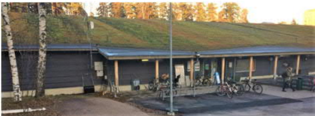
Scenic moss roof (est. 2015). The city of Helsinki demanded a new big sports hall to be covered by vegetation to scenically fit into a natural-like park. Moss was selected as the cover because the load support capacity of the roof was limited, and because there was an interest to test this new lightweight solution. The roof was designed using different substrate materials based on recycled or side products in different mixtures and proportions (e.g. compost, stone ash, soiled bark). The mosses clearly respond to the substrate so that the different test stripes are visible. Photo by S. Lehvävirta in 2019.
