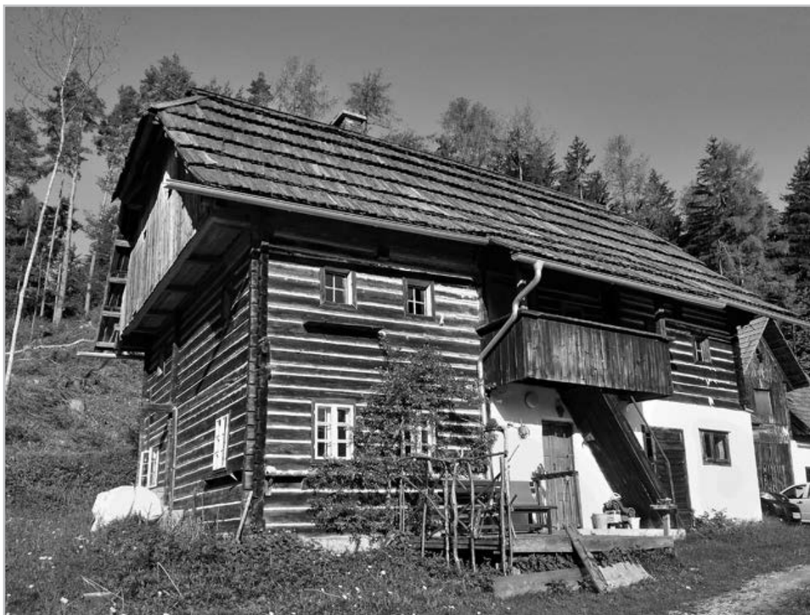
Figure 2: Wooden log-house in the Southern Austrian Alps from the early 18th century. Beside the stonewall-stable the building material is larch, harvested in the close surroundings. The house was part of a hammermill and is inhabited till present day (Photo E. Johann)
