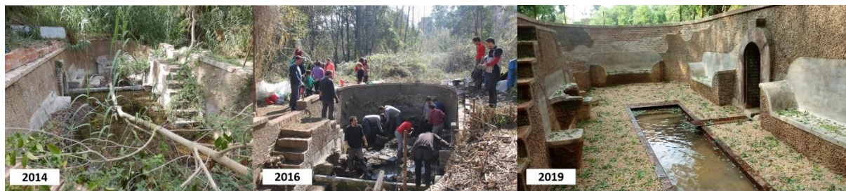
Figure 2. The spring of Can Moritz when first cleared of vegetation in 2014, during reconstruction in 2016 and after the restoration was completed in 2019 (pictures from Jordi Simó and Jordi Muntan).
