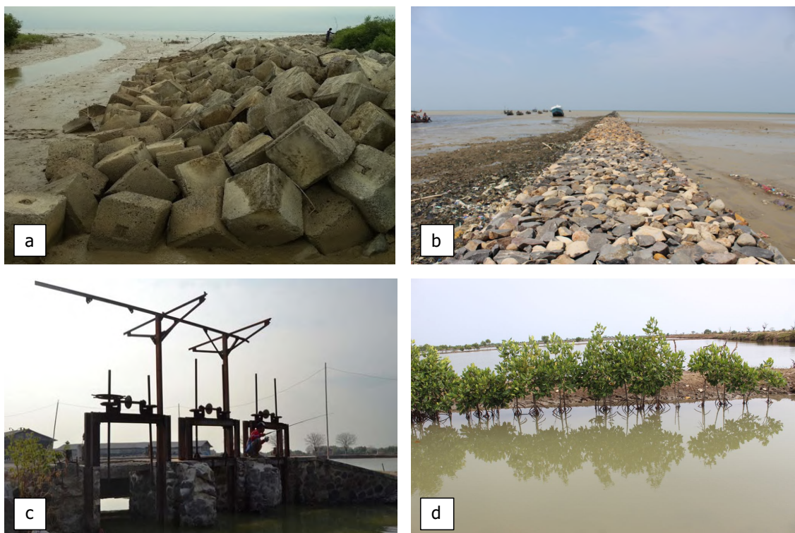
Figure 6.1. Coastal protection measures in a coastal area of Cirebon, including (a) breakwater (taken from Rawaaurip village); (b) groin structure in Gebang district; (c) water sluice gate (photo credit: radarcirebon.com, 2018); and mangrove plant surrounding the pond (captured in Suranenggala district)
