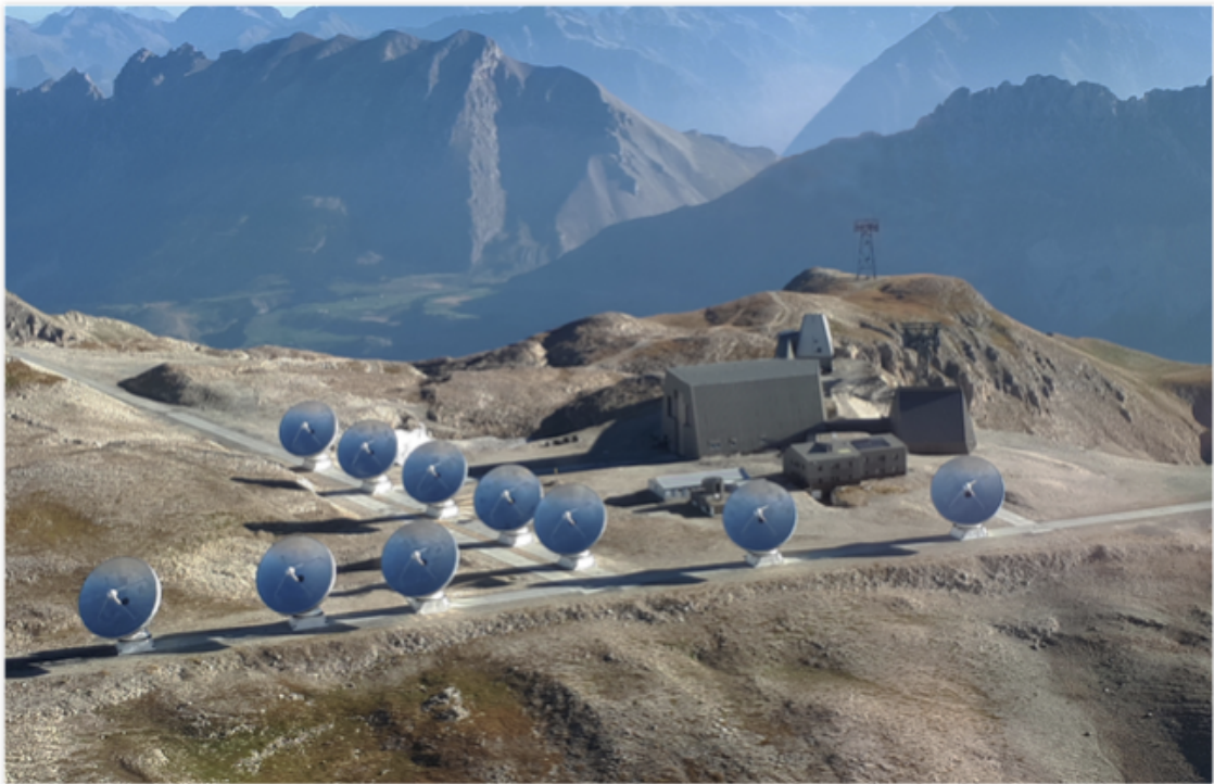
FIGURE 4.1: The NOEMA interferometer operated by IRAM, France. 15-m x 11 antennas are in operation in 2021, and 12 antennas are planned to be in operation. (Credit: IRAM)
