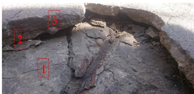
Fig. 2. The stratigraphic section of terrazzo pavement of Mohamed Ali Museum, 1) the concrete layer; 2) the underbed layer; 3) the topping terrazzo layer
