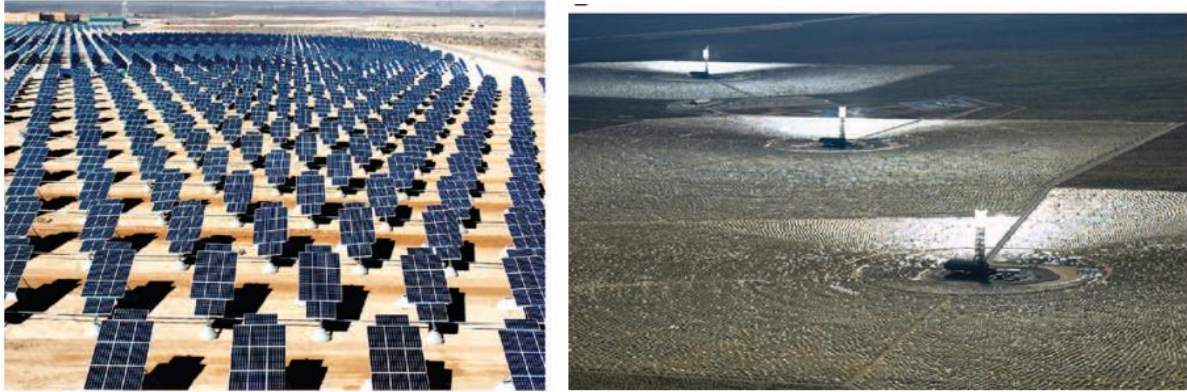
Figure 3: Installation of solar power plants: Photovoltaics (left) and Concentrated solar thermal (right) 15
