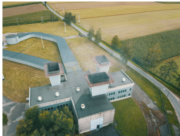
Figure 4.2: Mining ventilation facility Pniówek V. Drone-footage from Kud (2017).
