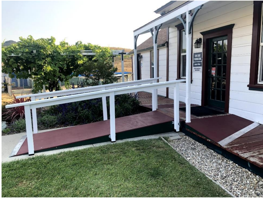
Figure 11: Side View of Completed Ramp
