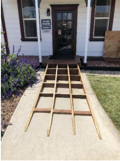
Figure 8: Frame of the Main Ramp
