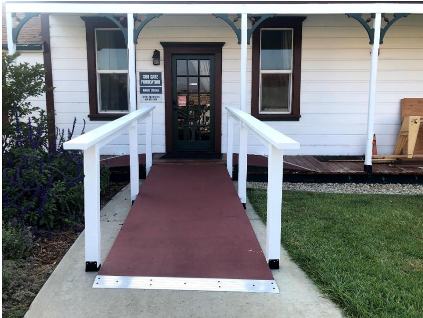
Figure 12: Front View of Completed Ramp
