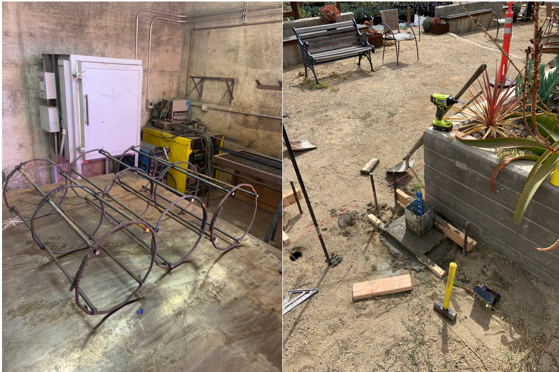
Image 8 & 9 – Rebar cages ready to set and post bases going in
