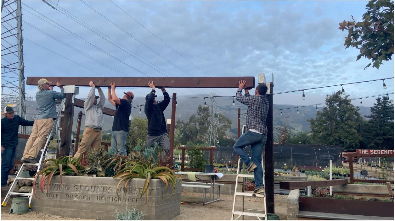
Image 13 & 14 – Team work to place the 6x8 beams
