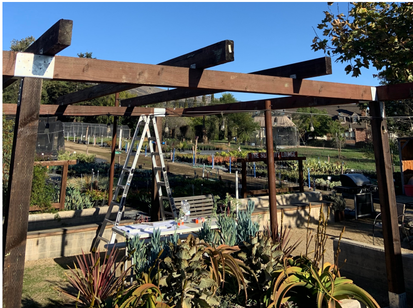
Image 19 – 4x8s fastened to 6x8s with Simpson ML24 angles. One on each side.
