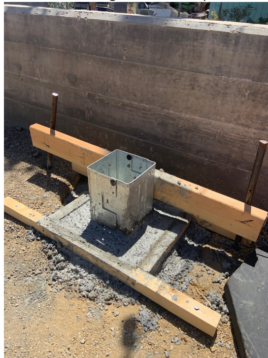
Image 11 – Post base installed and concrete cured
