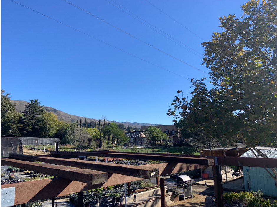
Image 18 – 4x8s moved into position ready to be aligned
