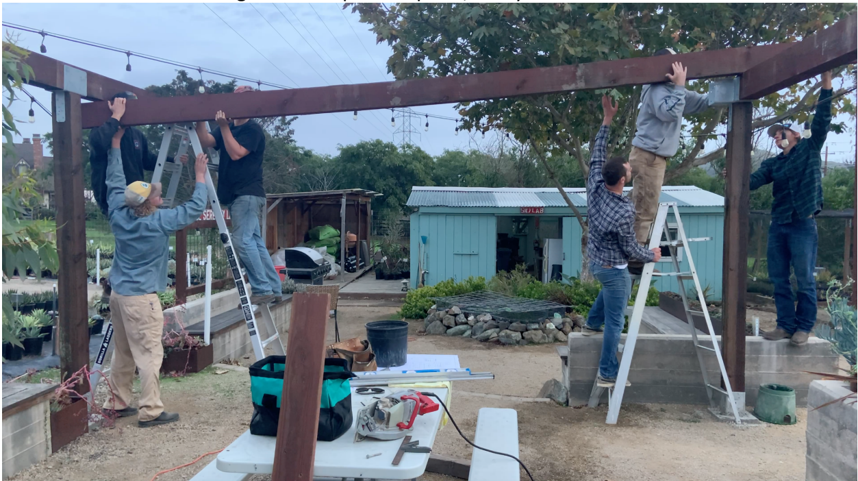
Image 12 – 6x6 posts in place, ready for 6x8 beams
