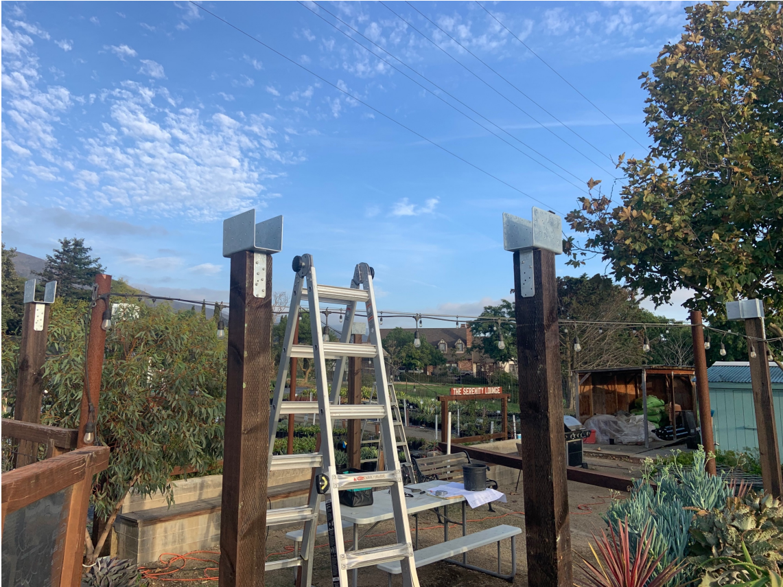
Image 12 – 6x6 posts in place, ready for 6x8 beams
