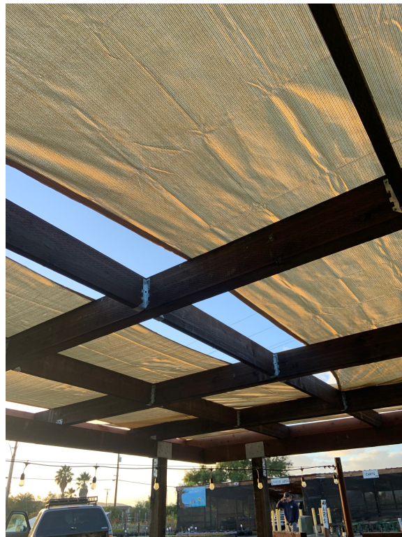
Image 26 – The structure from underneath
