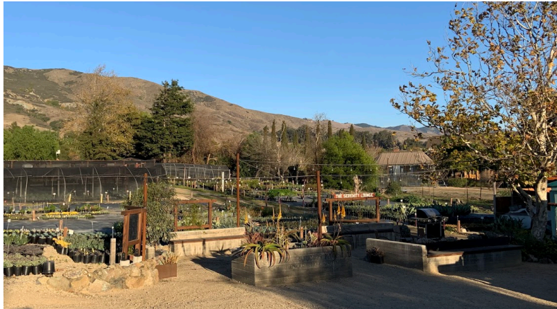
Image 1 – Site before construction (Winter 2021)
