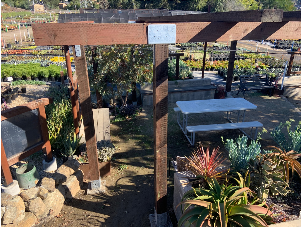
Image 16 – Post to beam connection
