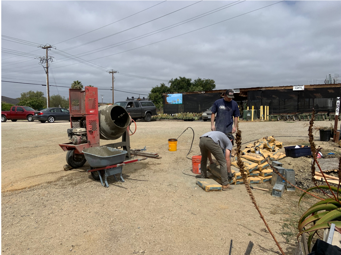
Image 10 - 50 90 lb. bags of concrete poured in one day
