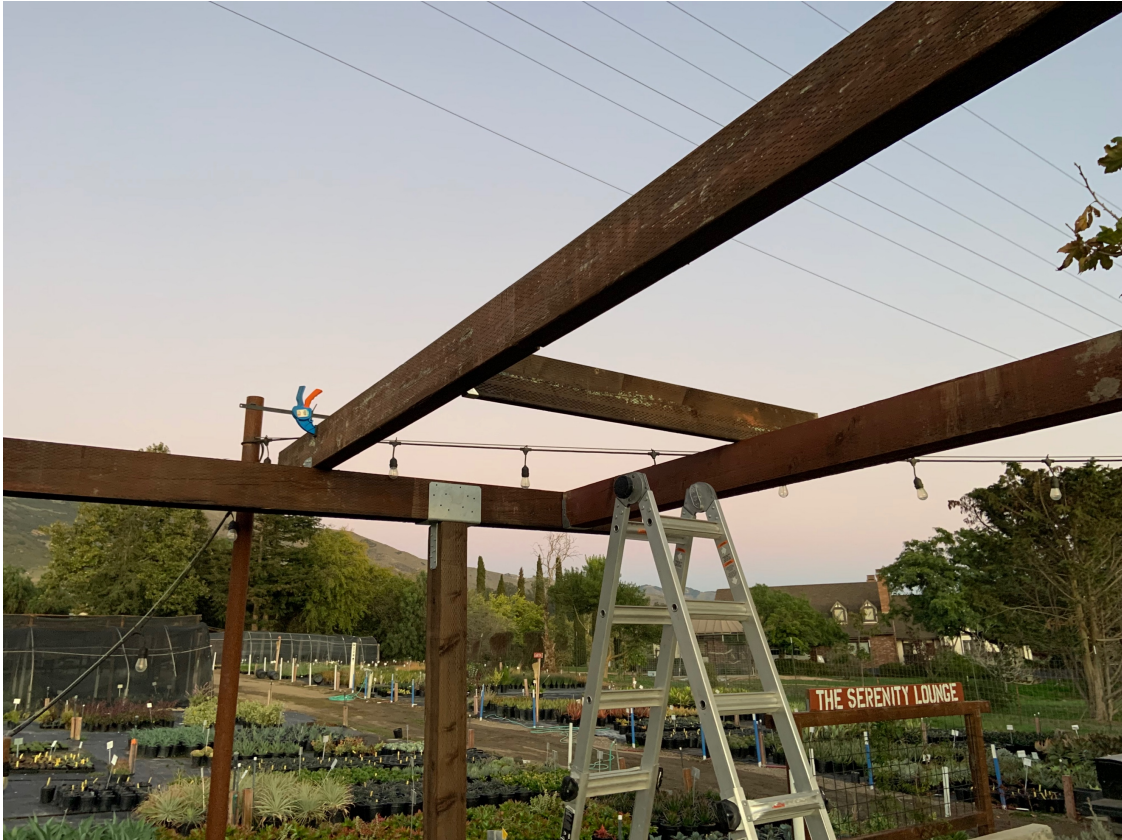
Image 20 – First perpendicular 2x8 installed.
