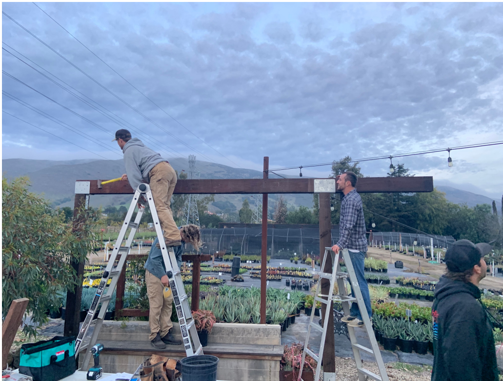
Image 15 – Hammering the beams into position
