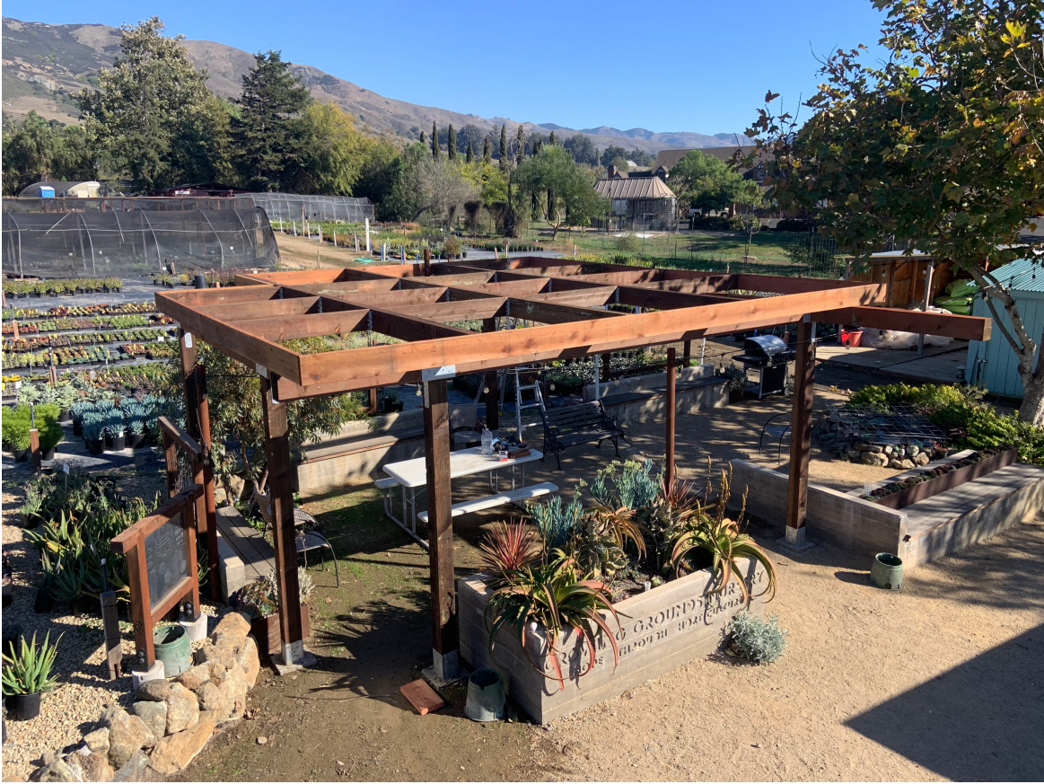
Image 22 – 2x8 redwood fascia installed. Ready for shade cloth
