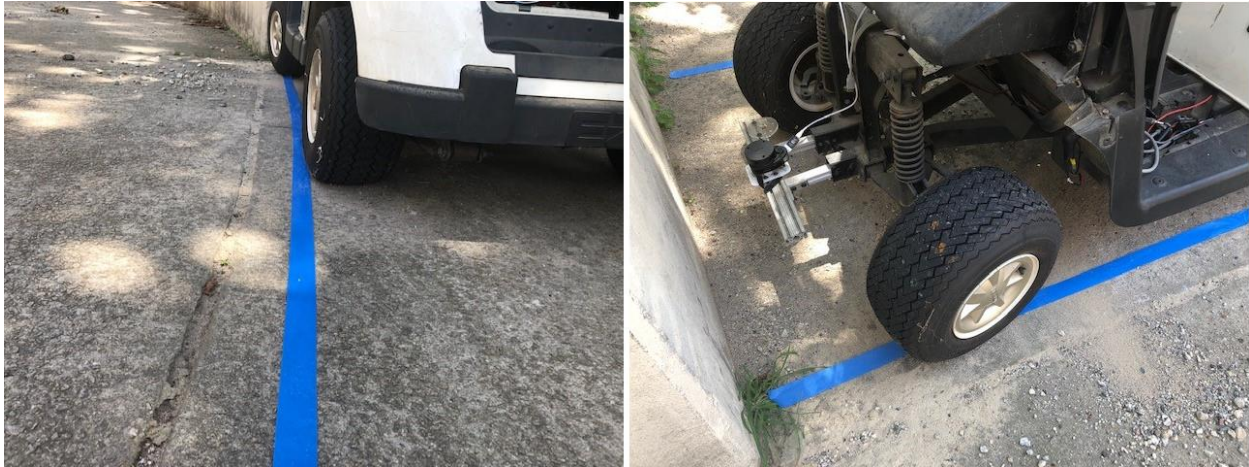
Figure 6-8: Example of a failed test
