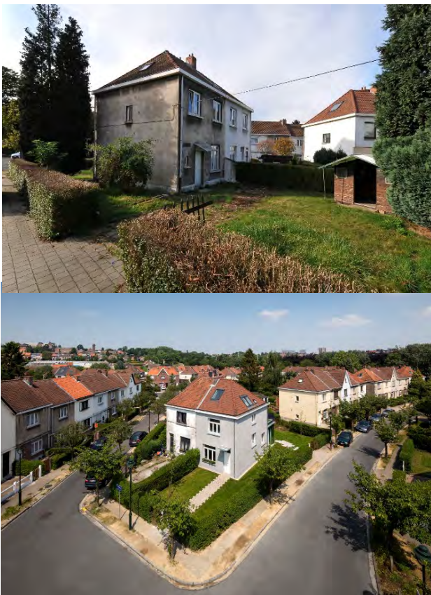
Figure 2 RenovActive prototype before and after renovation
