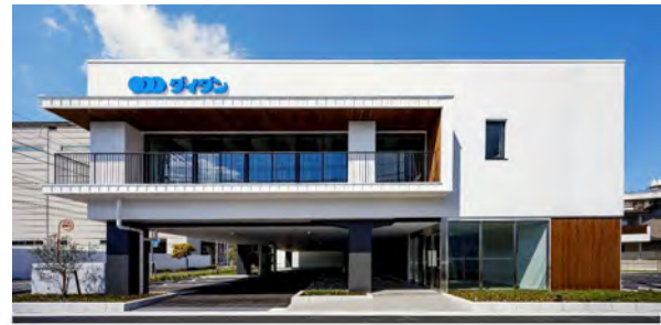
Figure 5. The ZEB office
