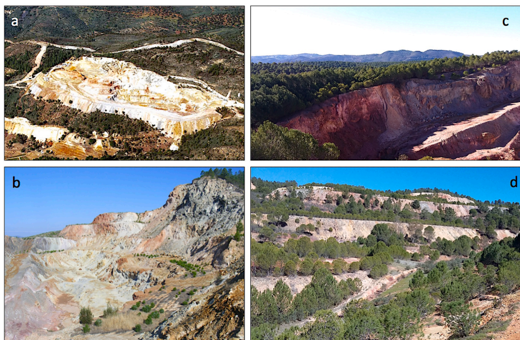
Fig. 4. Field pictures of the Poderosa mine site showing a chronosequence of the post-mining forest restoration: a) before land reclamation; b) shortly after the tree planting; c) open pit area 15 years after the land reclamation d) wastes dumps area 15 years after the land reclamation.
