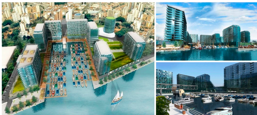
Figure 5. Visualizations of the Marina Dorćol according to the project of the company “Engel ma-rina Dorćol”. Source: beobuild.rs (accessed on 24 June 2021).
