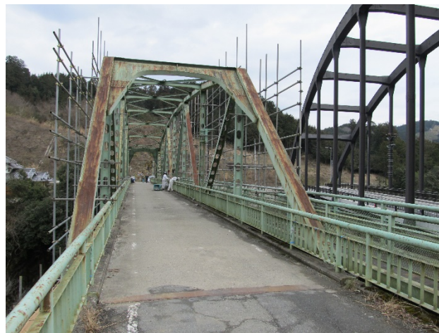
Figure 21 Overview of the bridge
