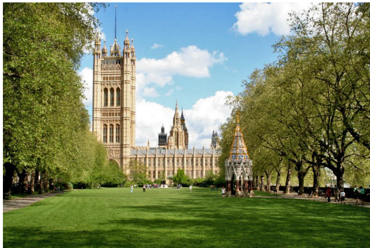
The Victoria Tower Gardens 204
