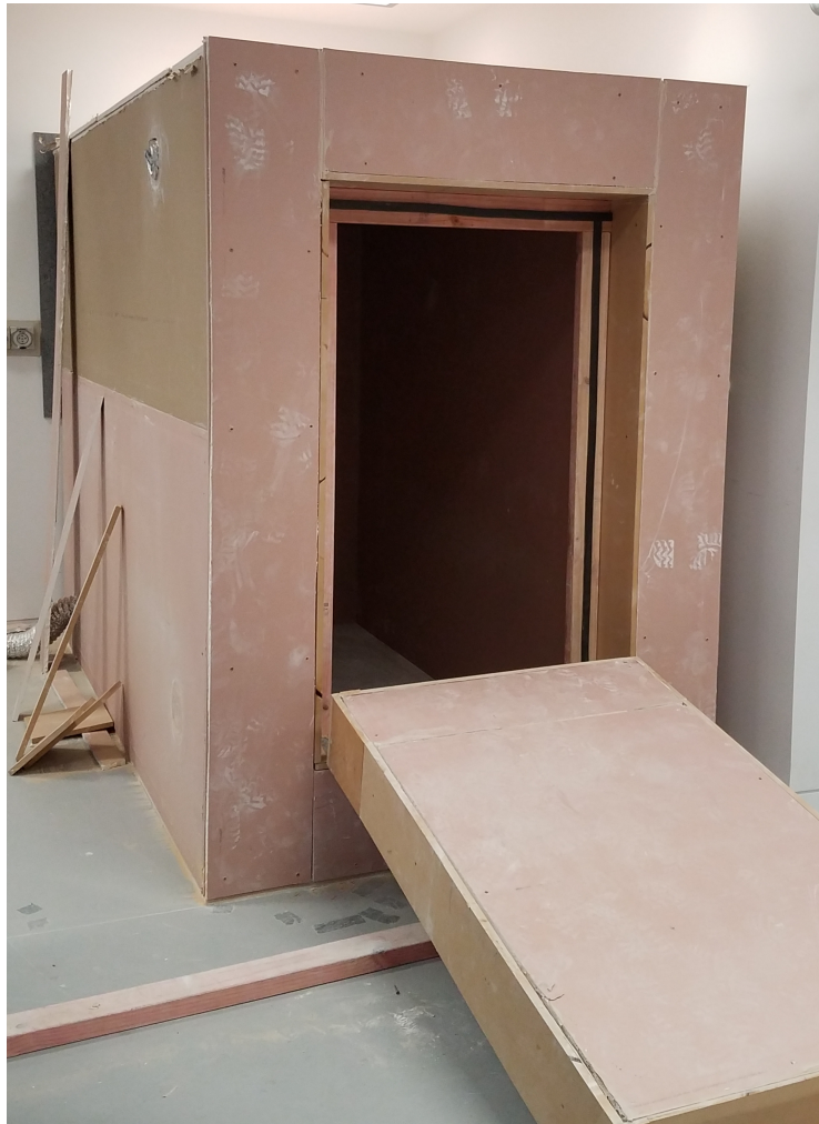
Figure 3.1: Testing chamber during construction.
