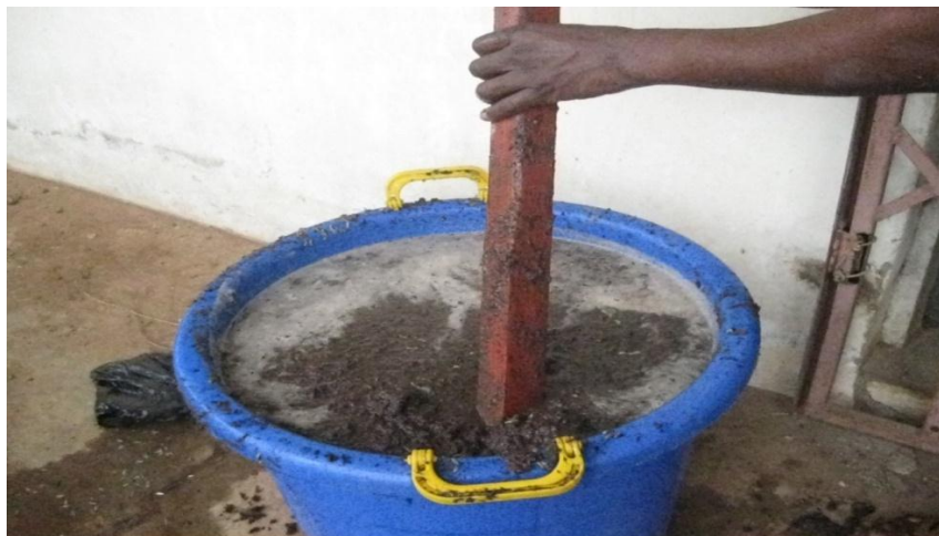
Plate 2: Slurry preparation in a pre-mix chamber
