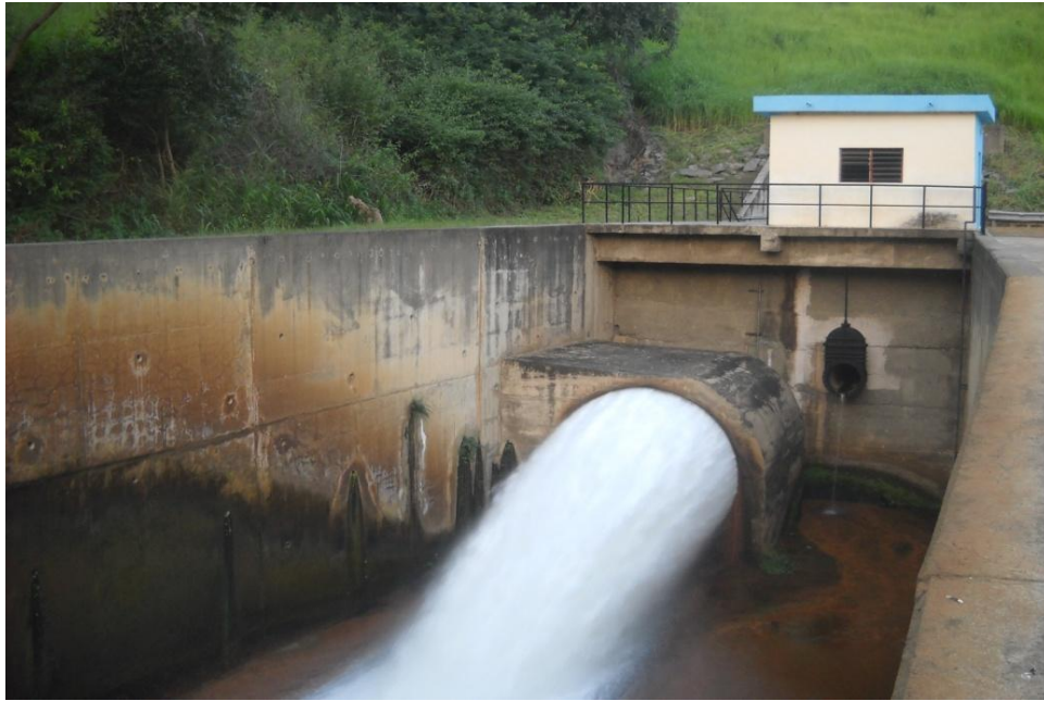
Figure 4. The water release outlet for Ikere gorge Dam.
