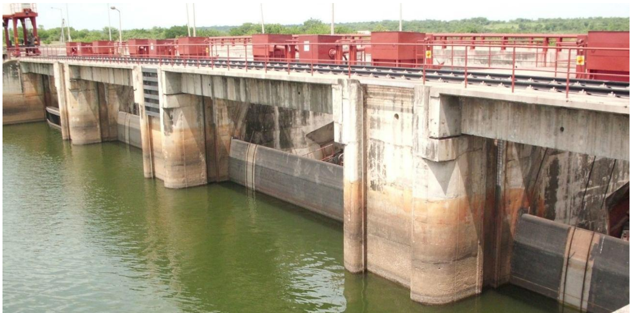
Figure 5. The spillway section of Oyan dam (Source: Olatunji, 2013).
