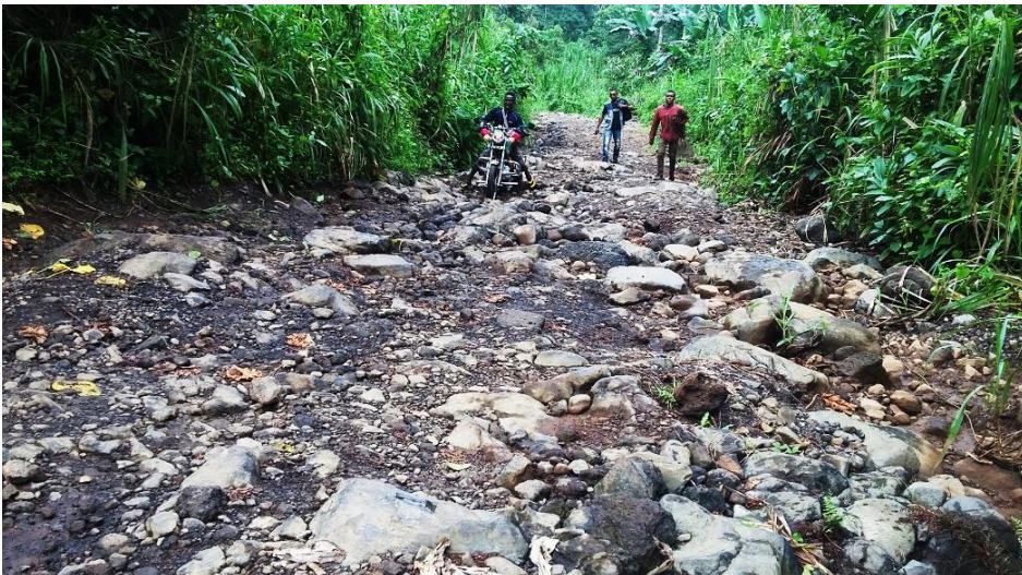
Figure 7. A continuation of the Muyuka-Munyenge earth road, in the Bomboko area (Field data 2017)
